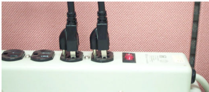
Figure 3.9: Power cord plugs should have same orientation in the socket/ 插座上电源线方向相同 / 插座上的電源線方向應相同
